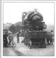
The contractors had a small railway for moving materials along the road during construction. The engine was a saddle tank, seen here as it arrived by road. It is rumoured that the remains of the engine are buried underneath the road near Brandhall. The lines do not look too secure, so it could easily have fallen from the track! The scene beyond the water tank shows well the countryside through which it was built. (Pictures: Sandwell Community History and Archives)
