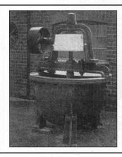
The first simple equipment used for making moulding powders at British Cyanides in 1925. Larger mixers and mills were required as production was increased. (Pictures: BIP)
