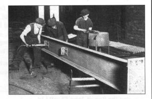
Pneumatic rivetting of beams and stantions. Hydraulic rivetting was also used.
