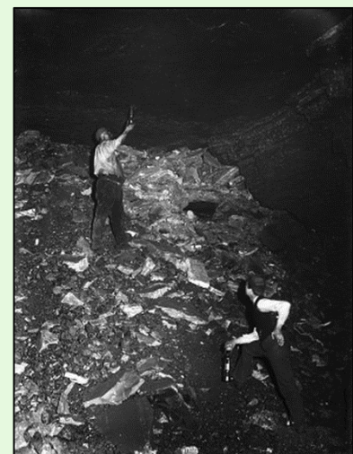
Testing for gas, Ramrod Colliery, 1890
